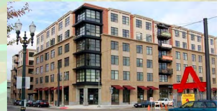
Sitka Apartments 6-story mixed use Portland, OR
